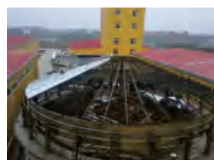
04 仓顶安装 Installation of silo top
