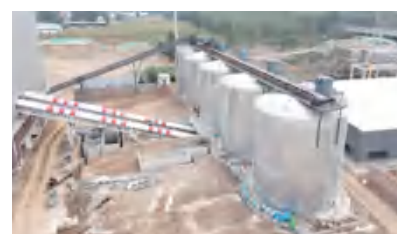
07 筒仓附属钢结构与设备安装 Installation of Silo Attached Steel Structure and Equipment
