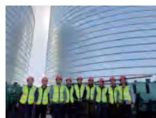
05 仓体卷制、顶升 Barrel volume system, lifting
