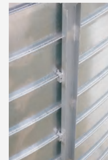
螺旋咬边仓壁成型图 The Forming chart of Spiral folding silo
